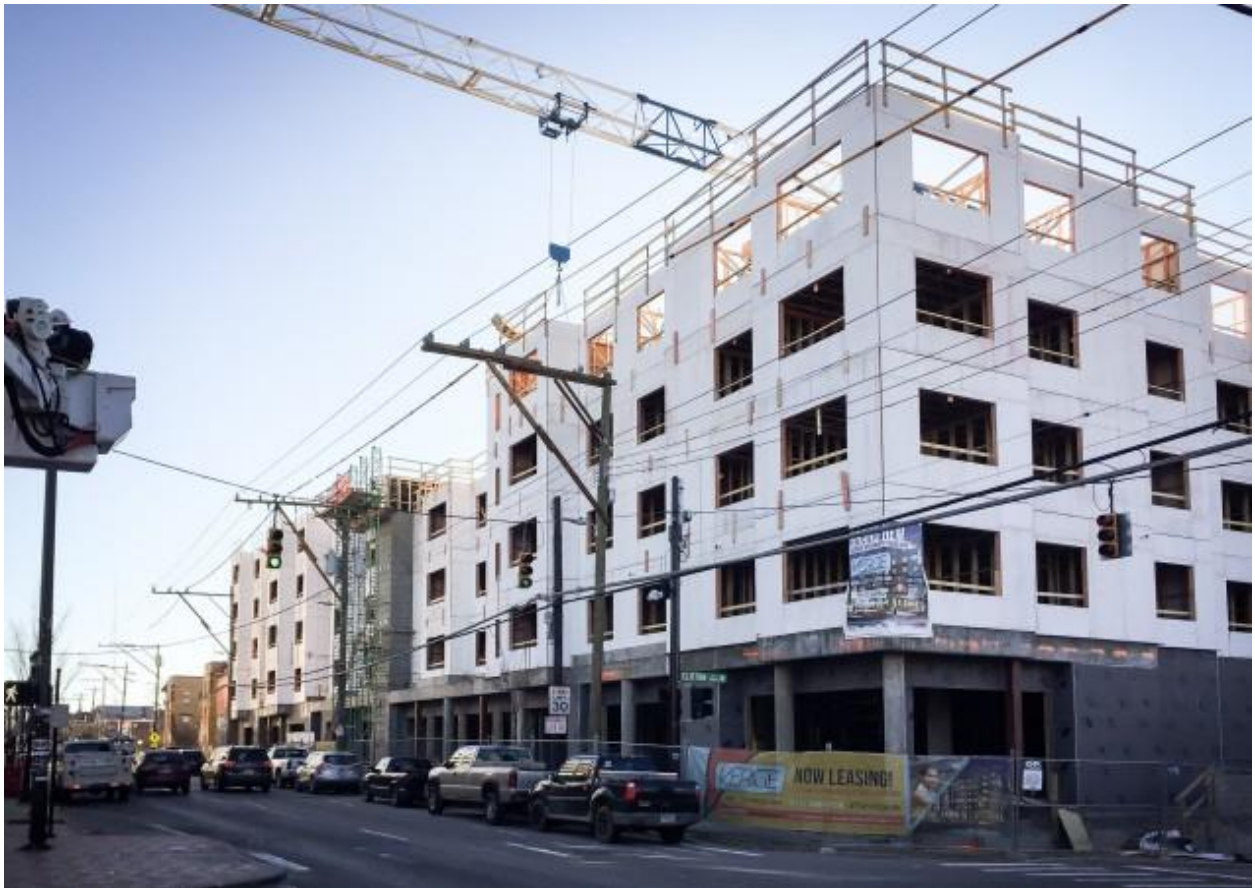
Fifth floor wood framing under construction.
