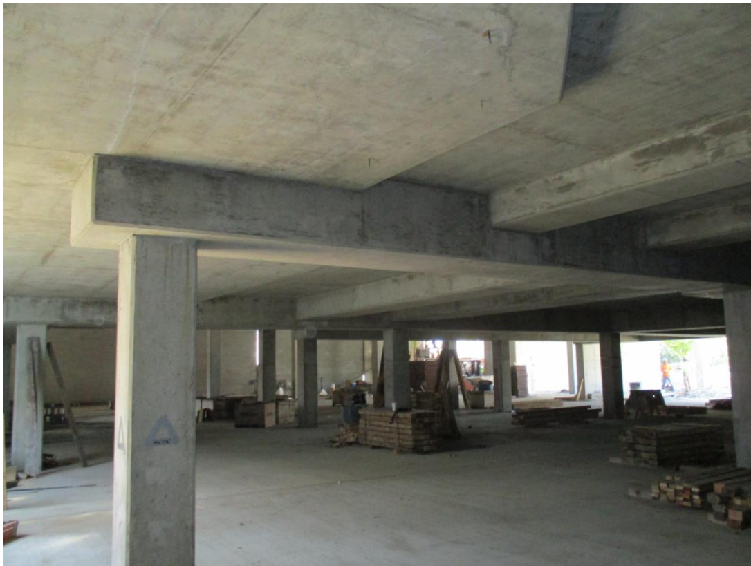
Transfer beams and slab folds below first floor in parking level.
