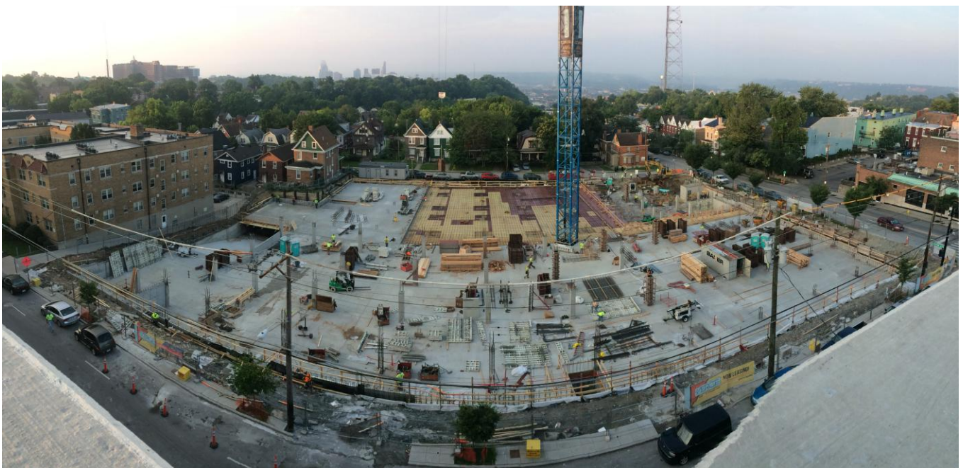
Parking Level P1 slab construction.
